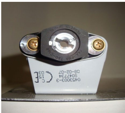
Cam Washers dialed full left of center
