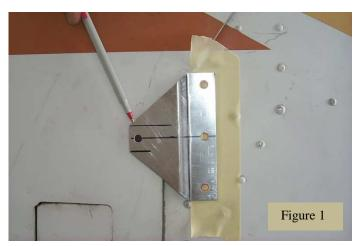
Sight template over each stud and mark holes onto tape. This important step will greatly enhance the alignment of each SK2003 mount at each location.
